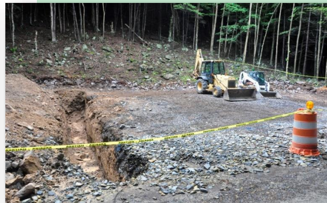
6-foot deep foundation trenches are dug.
