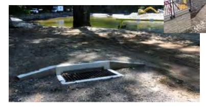
**To the left:** Repairs to the beach area included new drainage intended to prevent run-off from the road washing away the beach sand.
