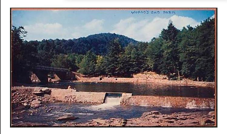
ABOVE: This old postcard shows the original dam built by the CCC in the 1930's. This dam was modified and replaced several times in the years since – most recently in 2021 when the dam was modified to incorporate additional spillways and walkways to allow easier access for park staff to maintain the dam and operate the spillways.
